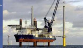
WTG Installation Vessel
