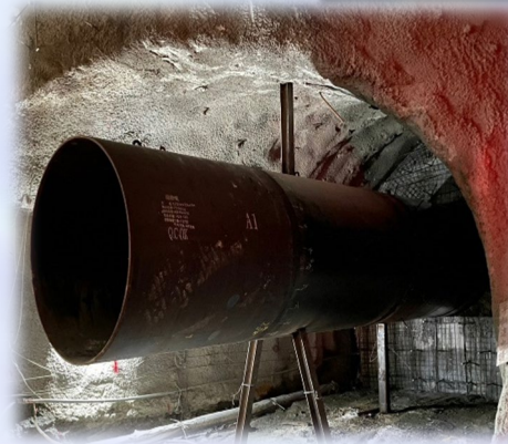
壓力鋼管銜接
