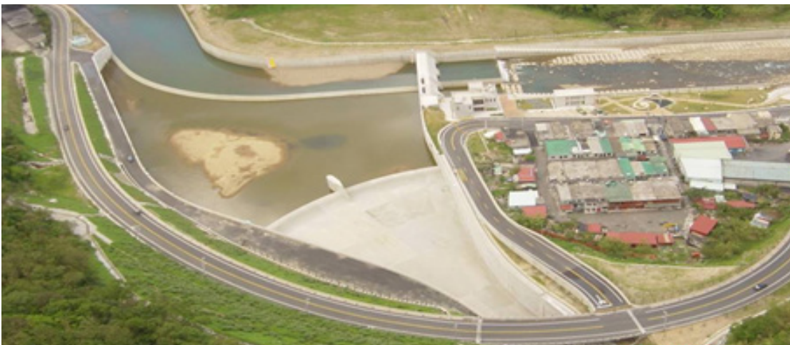
▲ Intake of Yuan-shan-tzu Diversion Channel
