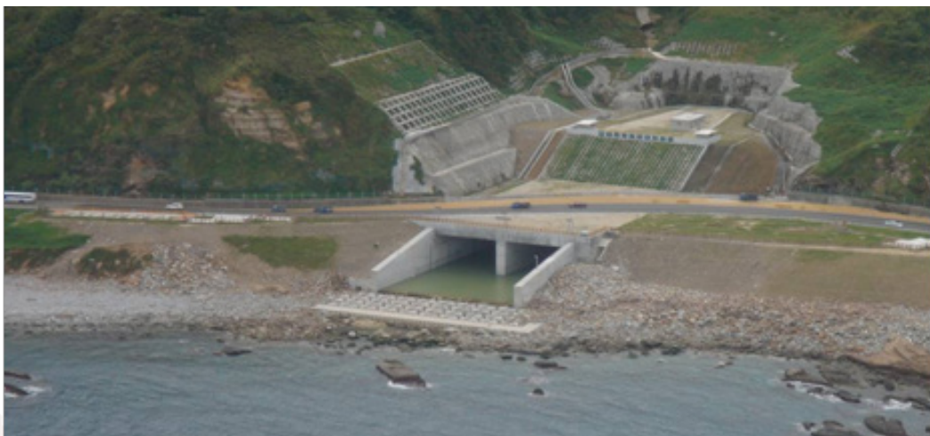
▲ Outlet located on Shoreline
