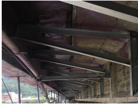
(A) 橋面側撐補強
