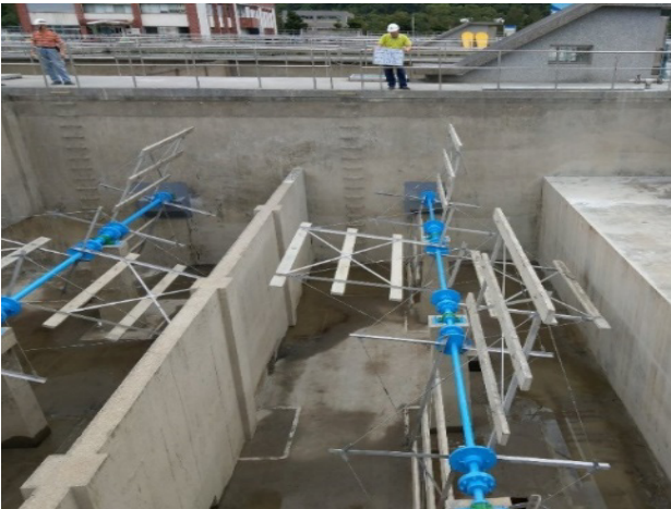
▲ Mixers and scrapers replacement in water purification plant
