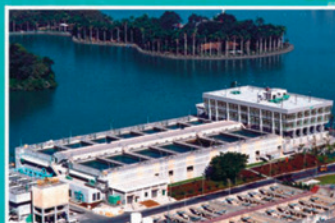
澄清湖高級淨水處理設備工程 Chenchin Lake Advanced Water Treatment Plant
