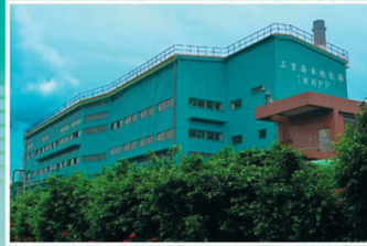
工業廢水純化場 Industrial Waste Water Purification Plant
