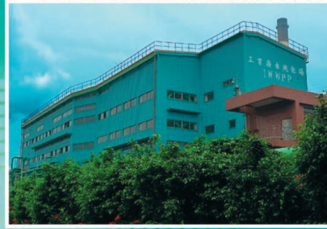
工業廢水純化場 Industrial Waste Water Purification Plant
